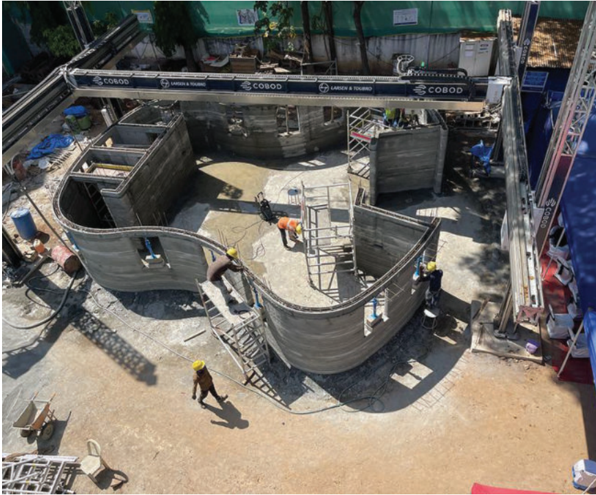
Next big thing: 3D concrete printing equipment on the construction site of the new Halasuru post office. K. MURALI KUMAR
